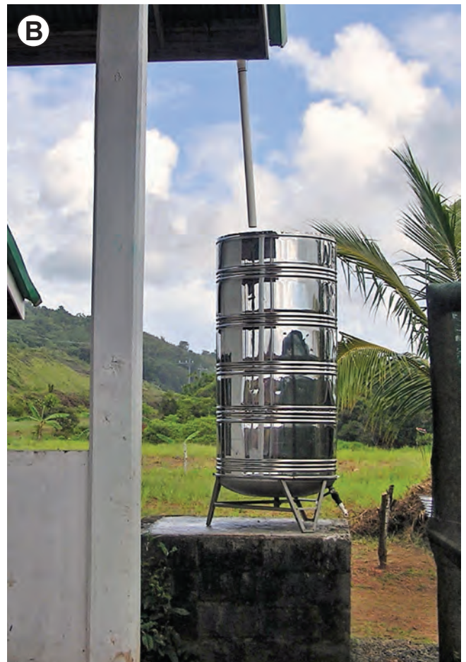
Figure 2.13 —Planning for local environmental conditions and for risk is essential during the process of nursery design. This nursery in Guam uses natural windbreaks to reduce water use and add protection to the nursery site (A); this nursery in Palau catches rainwater as a backup water supply (B). Photo A by Tara Luna, and photo B by George Hernández.
