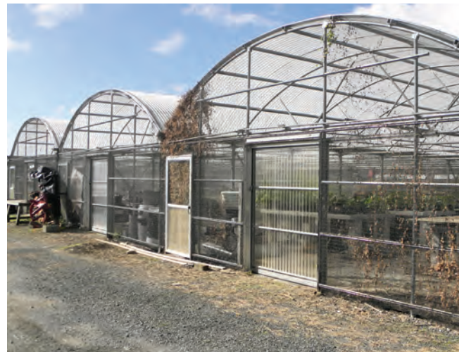
Figure 5.9 —Greenhouses are covered with transparent coverings such as plastic sheeting or hard plastic panels to maximize the amount of sunlight reaching the crop. Photo by Brian F. Daley.
