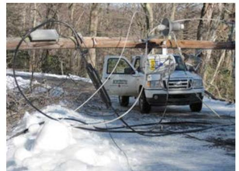
Power lines brought down by broken trees pose a serious electrical hazard to the public and workers, as well as a blocking transportation for emergency vehicles. Photo courtesy of Asplundh.
